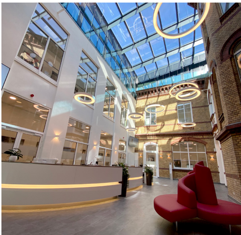
As part of the core renovation of the old hospital, the combination of tradition and modernity was achieved architecturally (photo: Rayk Weber)
